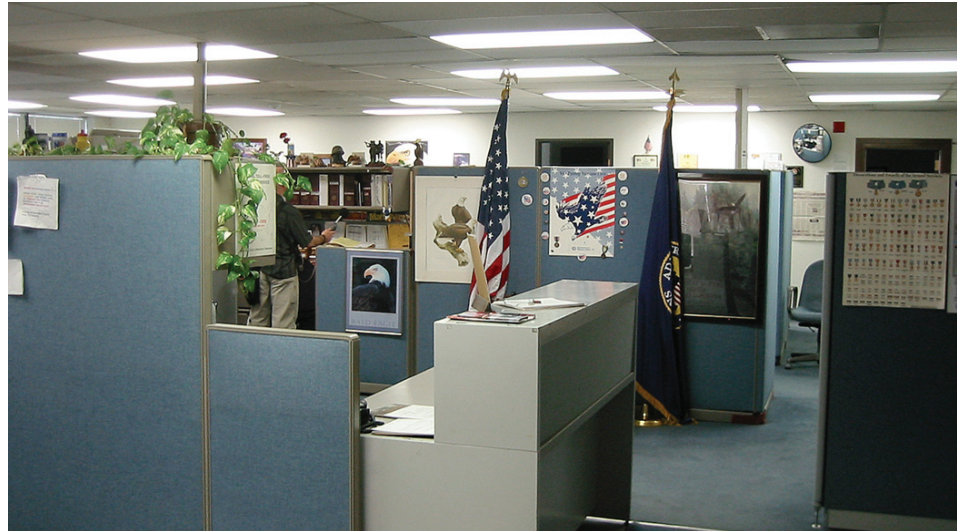
Ceiling lights with flush lens covers create direct and reflected glare for computer work.
